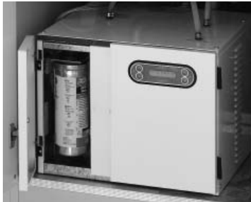
Hydotap undersink assembly. The appliance must be placed in a horizontal position, as shown above.
